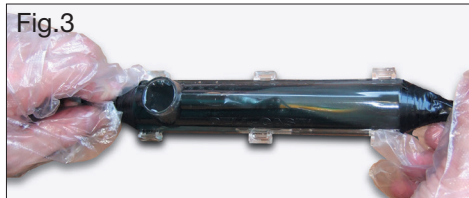
Fig. 3: Cast the shell with prepared casting resin
