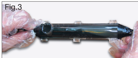
Fig. 3: Cast the shell with prepared casting resin
