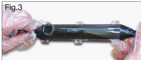
Fig. 3: Cast the shell with prepared casting resin
